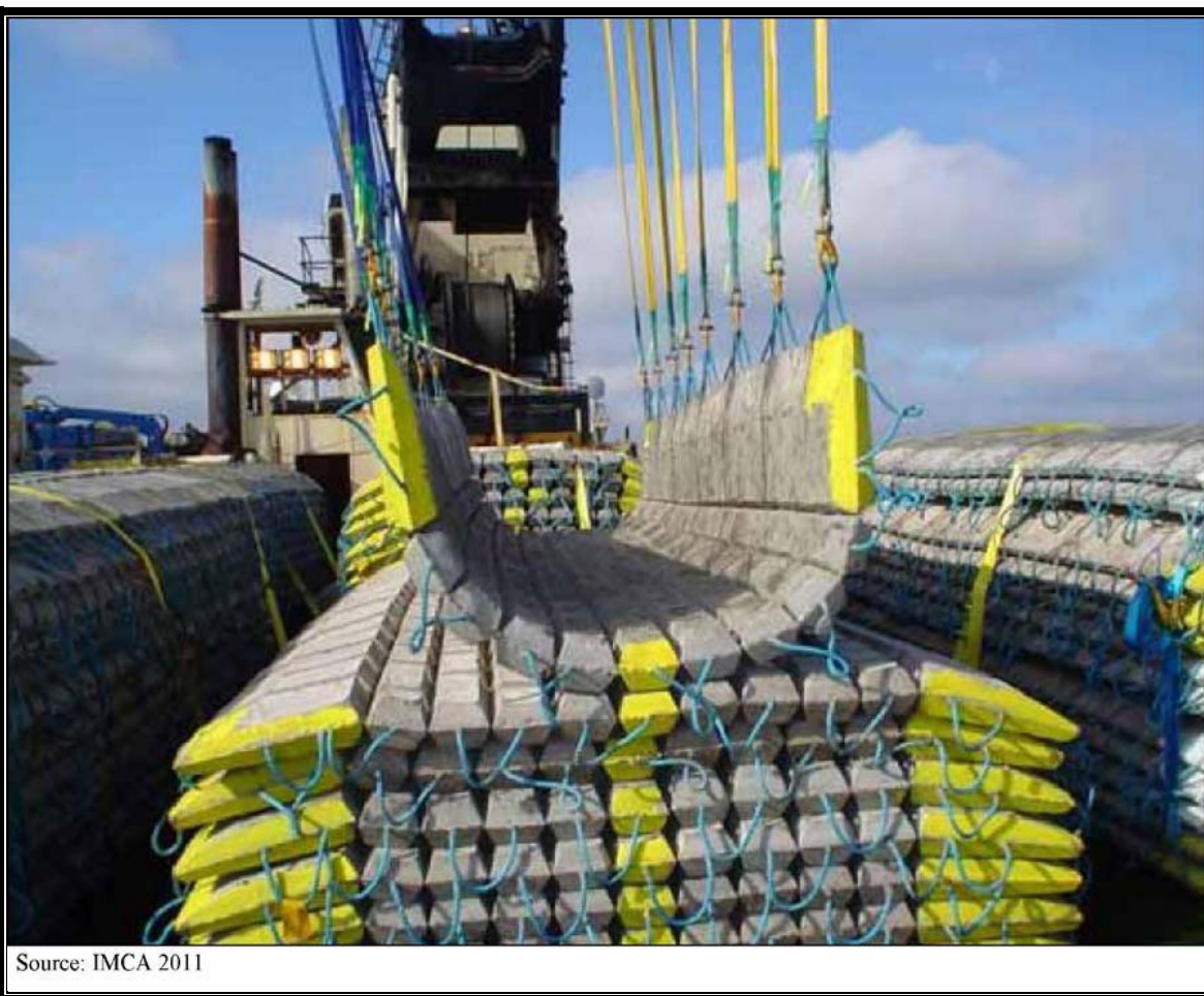
FIGURE 2-5 TYPICAL ARTICULATED CONCRETE MATS
